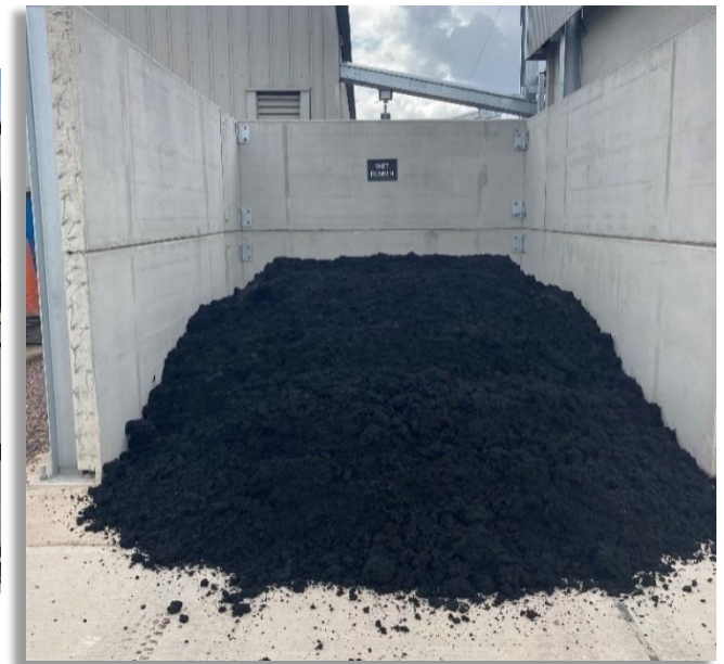
Fig 6. Sludge storage bunker
