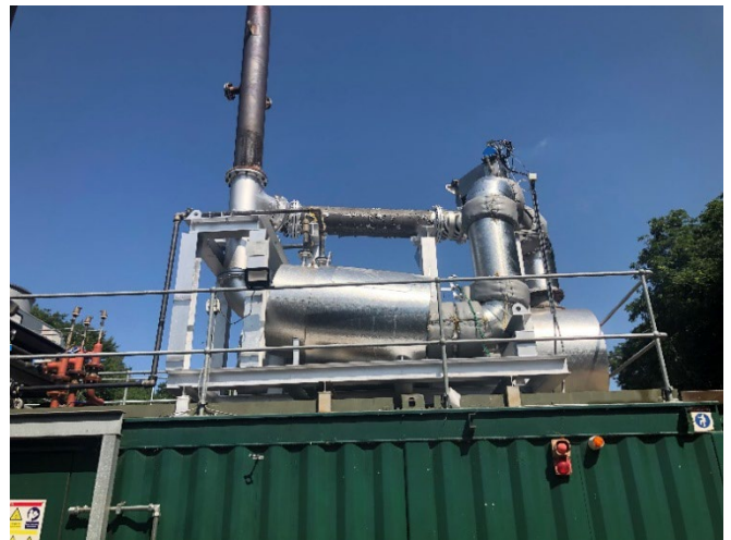
Figure 4 Waste heat recovery
