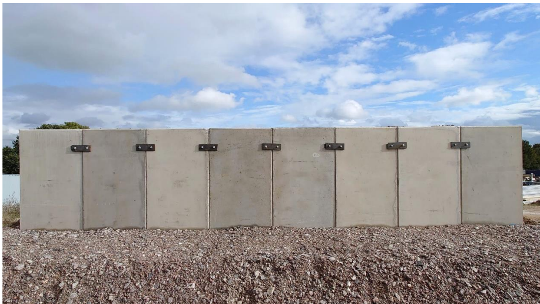
Figure 5 - Completed demonstration at the HS2 South Portal site
