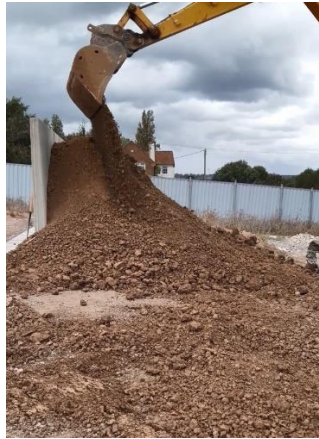
Figure 4 - Sequence of backfilling retaining walls with sulphated soil (clockwise from top left)
