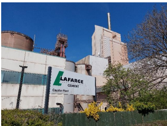
Figure 4: Exterior of Caudon Cement Works
