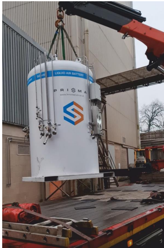
Figure 7: The installation of PRISMA at Caudon
