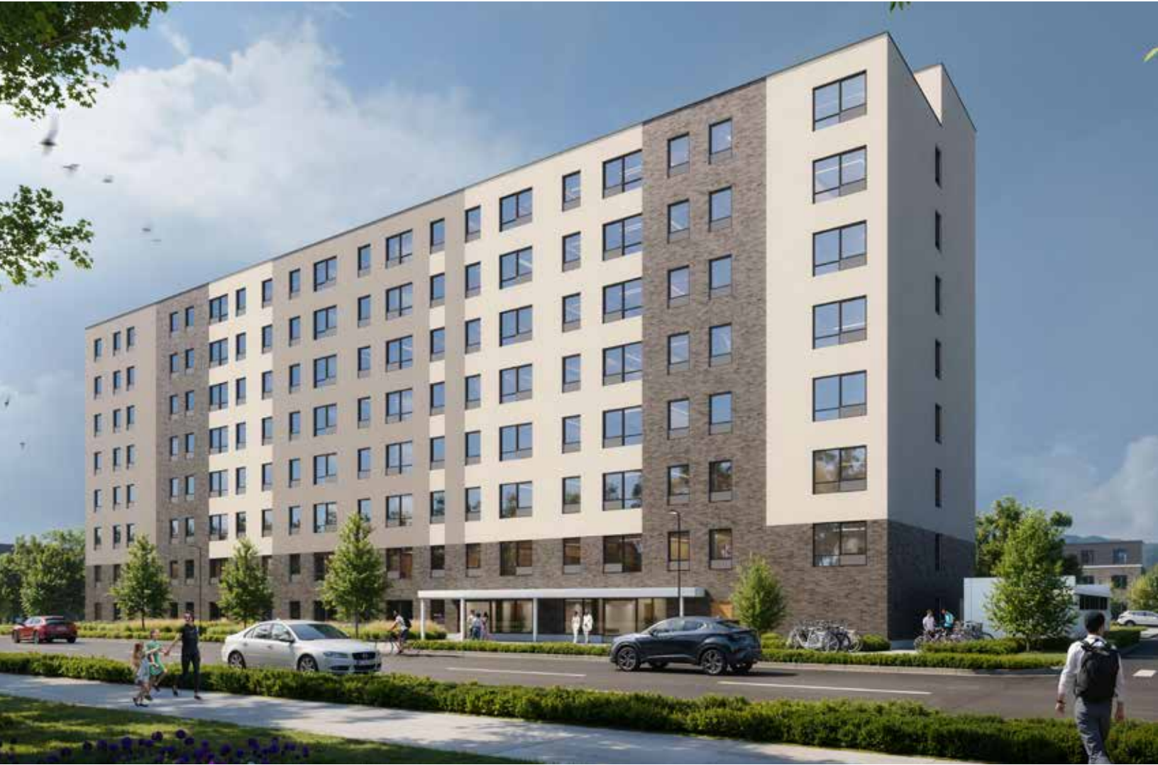
8-storey building with EIFS and brick facade
