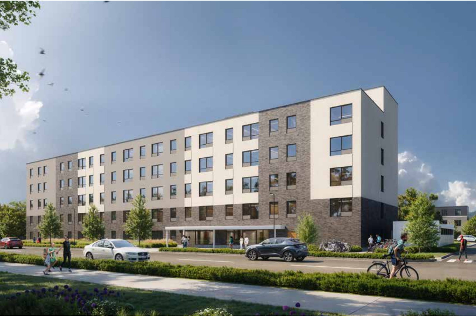
5-storey building with EIFS and brick facade
