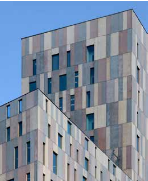
Exterior Insulation and Finish Systems (EIFS).
