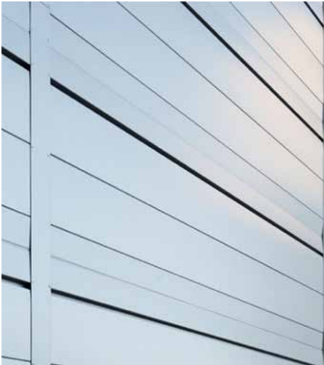
Metal siding in white tones (above and below windows).
