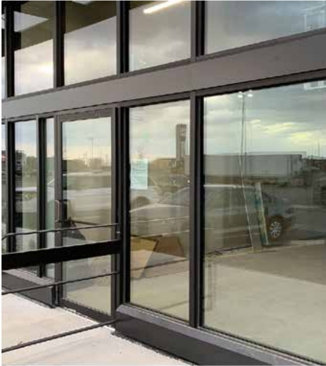
Storefront curtainwall at entry and shared amenities
